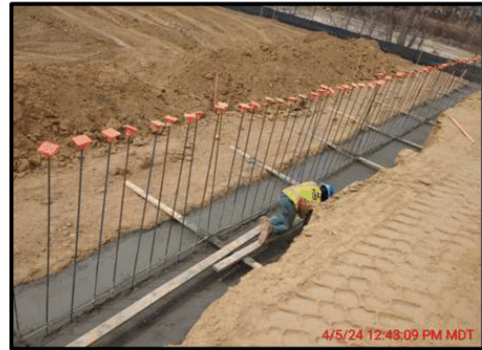
Building 9 Retaining Wall Footing
