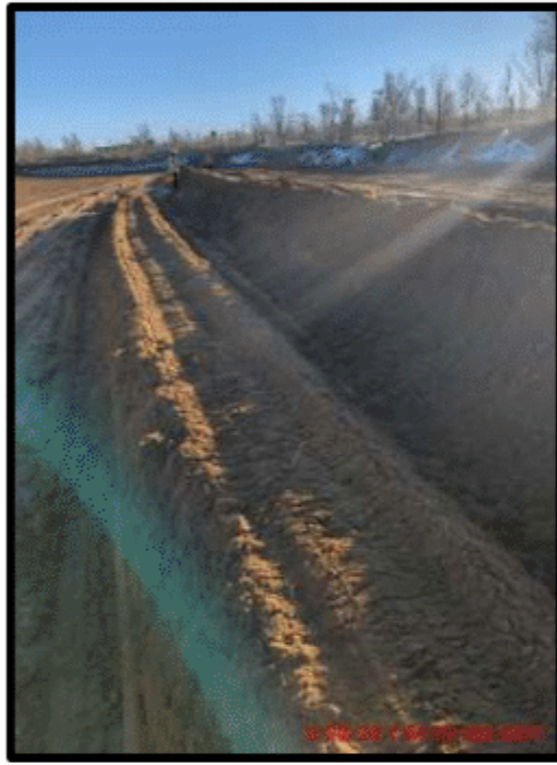
Building 9 Retaining Wall Bench Preparation
